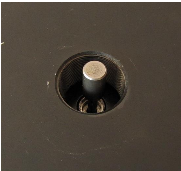
Placing “the puller” in the bearing casing
